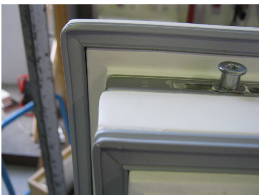
Fig. 2 Middle gasket and internal rebate seal, corner design
