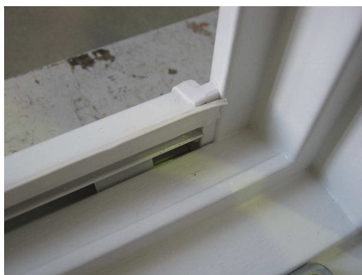
Fig. 3 Drip rail, connection detail
