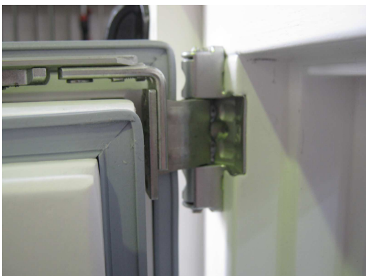
Fig. 4 Tilt mechanism pivot, seen from rebate
