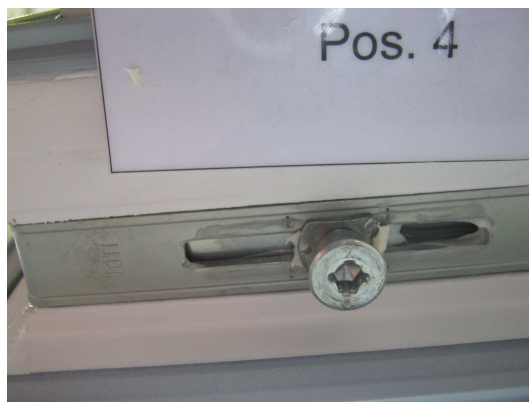
Fig. 14 Locking situation casement Pos.4
