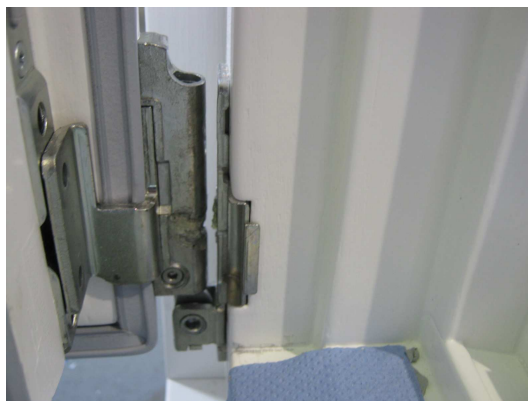
Fig. 5 Corner pivot, seen from rebate
